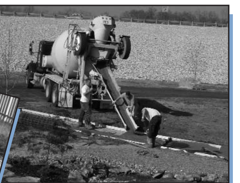
Above: Concrete for the pathways is poured.
