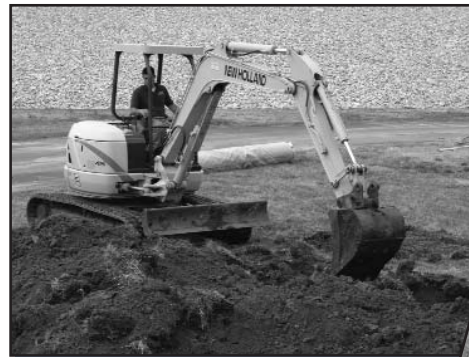
Above: Workers break ground on the garden.
